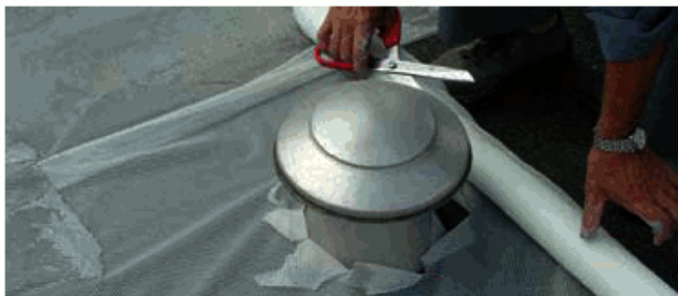
Extra mechanical strength can be obtained by using reinforcement fleeces.
