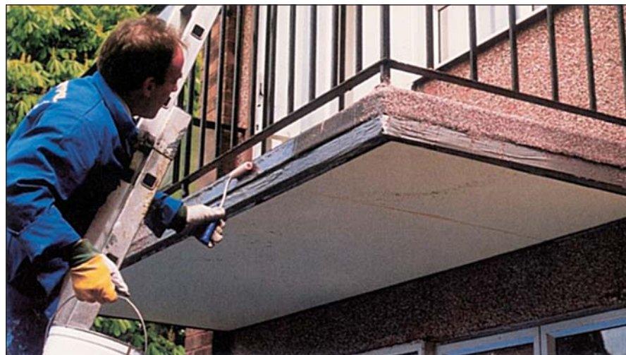
Coating the edges with Quartzdek transparent resin and scattering in the Quartz granules.
