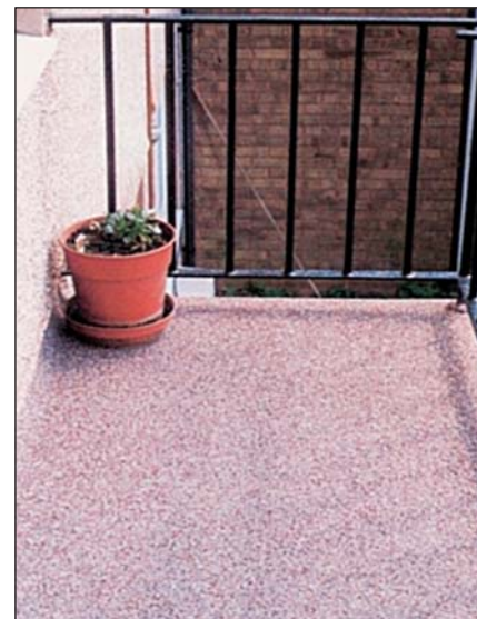
Final coat of Quartzdek transparent resin sandwiches in the Quartz granules and transformation is complete!
