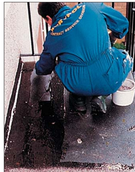
Applying Quartzdek transparent resin base coat by mohair roller to the asphalt floor.
