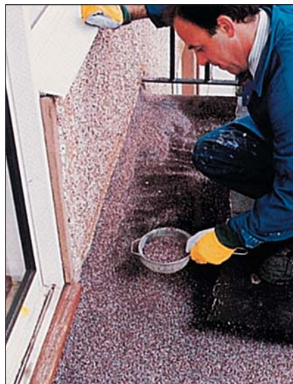
Scattering the Quartz granules onto the wet Quartzdek transparent resin base coat using a strainer.
