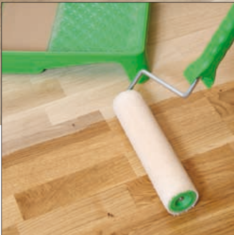
First coat applied with a Floor brush or Microfibre Roller
