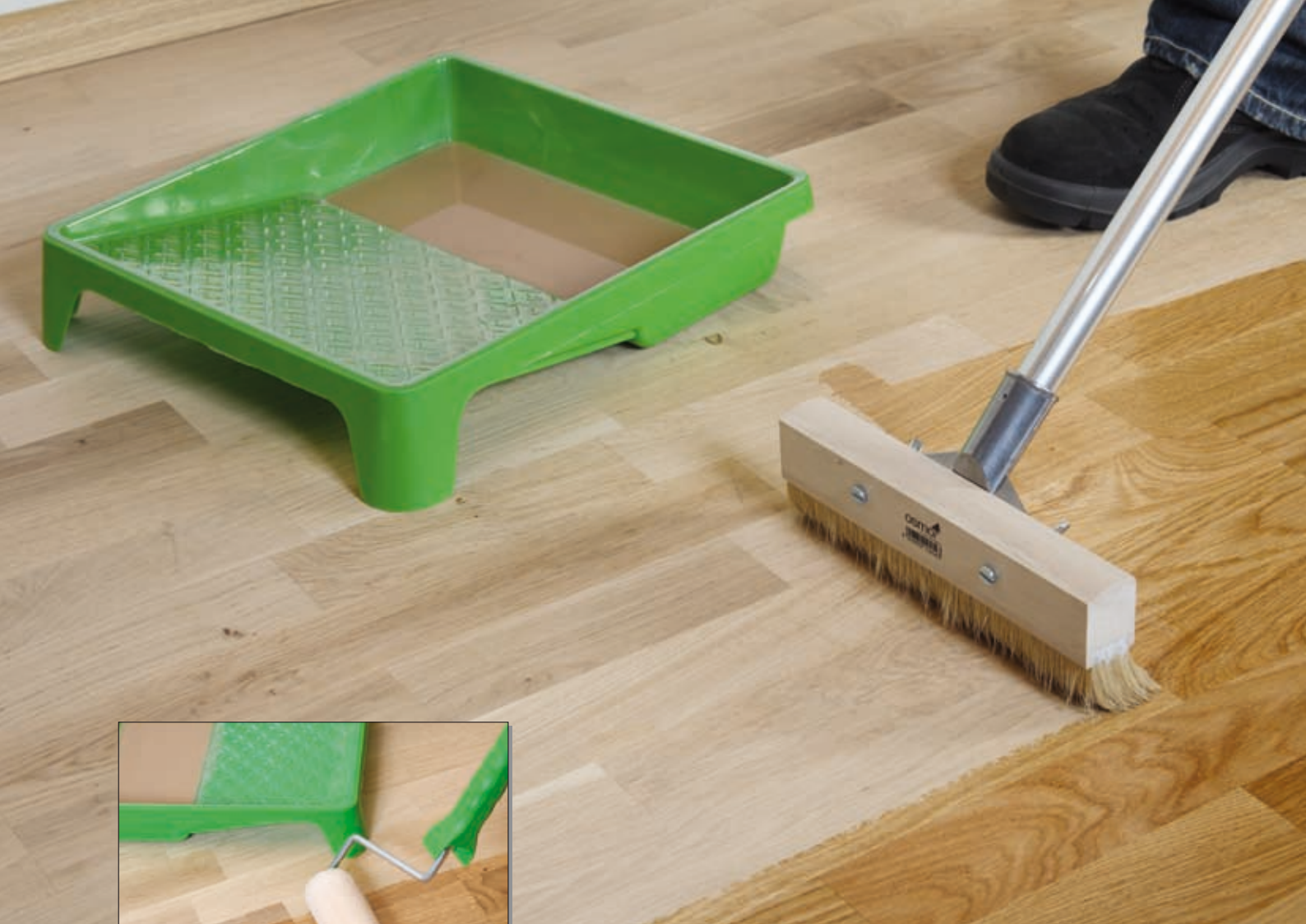
First coat applied with a Floor brush or Microfibre Roller
