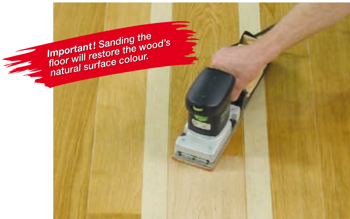
21) Even sanding of the damaged surface
