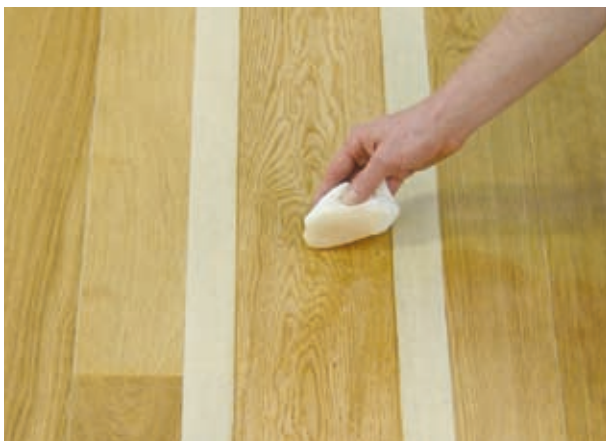
23) Thin application of Osmo Polyx ® -Oil after leaving the first coat to dry thoroughly
