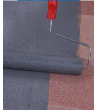
Application of Eco Prim Grip by roller on existing terrazzo flooring
