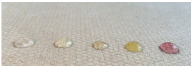
Protected Concrete Surface
