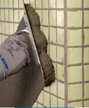
Applying Planitop 200 on glass mosaic
