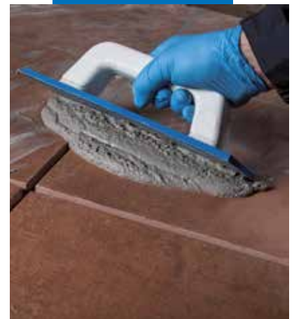
Grouting tiles with Ultracolor Plus
