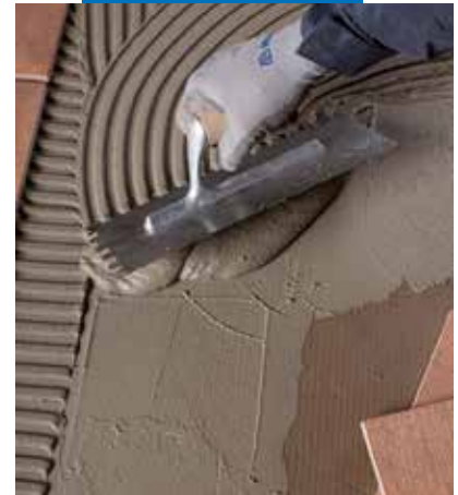
Bonding tiles with Elastorapid
