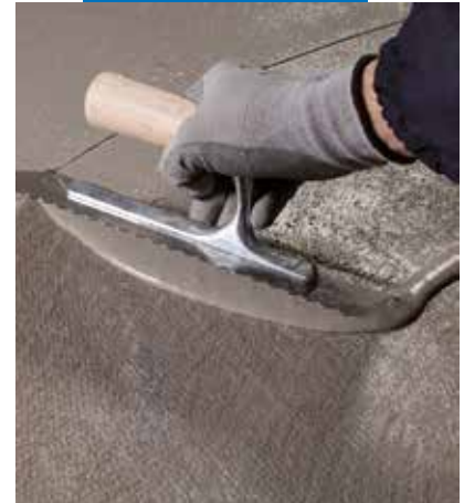
The second layer of Mapelastik Turbo over the first layer reinforced with Mapetex Sel
