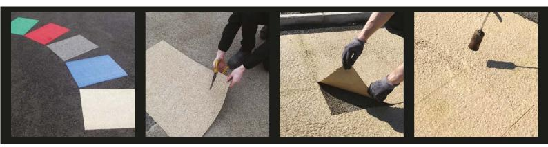
Centrecoat Thermoplastic Anti Slip Sheeting are a preformulated thermoplastic sheet, produced with high quality resin binders, selected aggregates and a pre- embedded anti-skid coating including bauxtite. Supplied in 0.6m2 sheets, this product adheres to the existing surface by gas torch heating.
