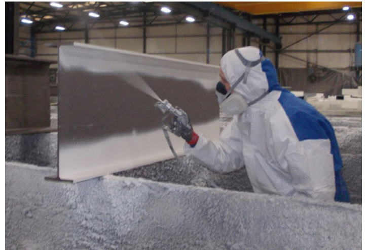
Interchar® 2090 being applied to an I-section
