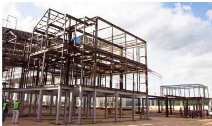
A modular construction project due to the isolated location, with fabrication and application in Thailand
