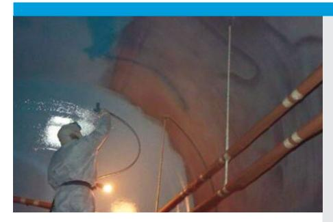
Phenoline 353 is a two-coat lining system with extraordinary overall chemical resistance and versatility. This product has a unique blend of resin chemistries that make it highly resistant to a variety of aggressive cargos. Phenoline 353 LT has additional low-temperature cure capability.
