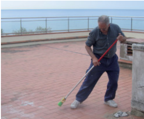
Cleaning a substrate before applying Aquaflex Roof
