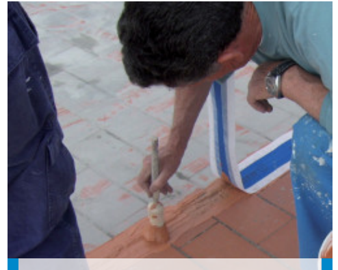
Waterproofing a distribution joint with Mapeband fixed in place with Aquaflex Roof
