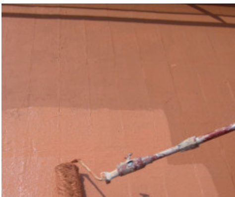
Application of Aquaflex Roof with a long-piled roller
