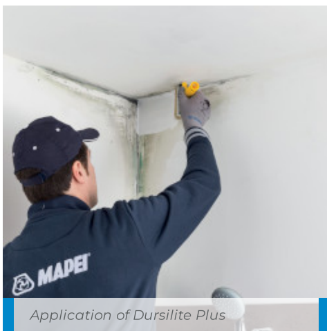
Surface sanitised by applying Dursilite Plus
