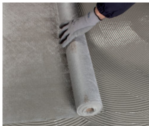
Placing Mapenet Sel on the first layer of Mapelastastic Turbo while wet
