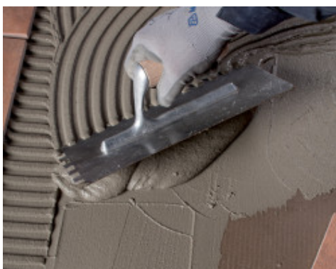
Placing Mapenet 150 on the first layer of Mapelastastic Turbo while wet
