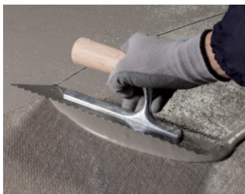
The second layer of Mapelastastic Turbo over the first layer reinforced with Mapetex Sel
