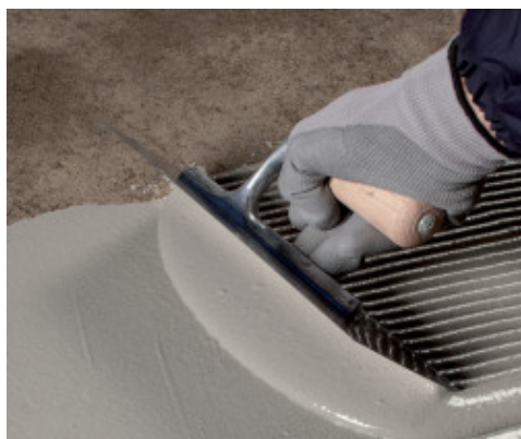
Application of the first layer of Mapelastastic Turbo
