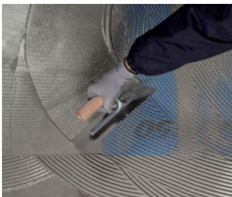
Placing Mapenet 150 on the first layer of Mapelastastic Turbo while wet
