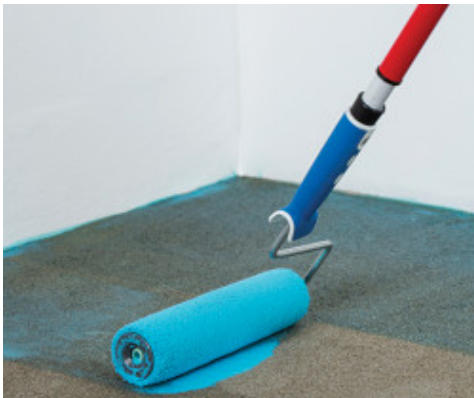
First coat application of Mapeproof Primer
