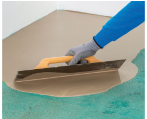
Self-levelling compound application on Mapeproof Primer
