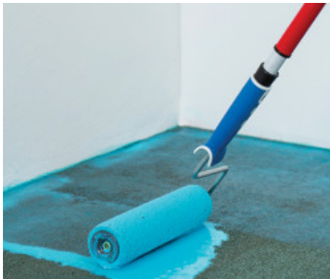
Second coat application of Mapeproof Primer
