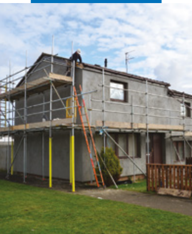
Work on a EWI housing project using Mapetherm AR1 GG
