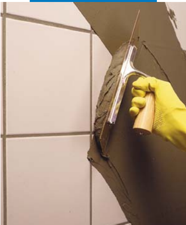
Smoothing an existing wall covering with Planipatch
