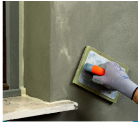
Floating the surface of Planitop 210
