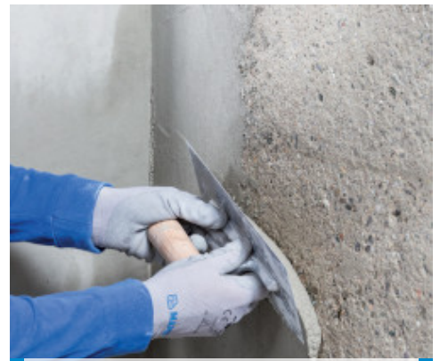
Applying Planitop Smooth & Repair R4 with a trowel
