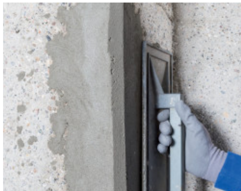
Floating the surface of Planitop Smooth & Repair R4 to create a smooth finish
