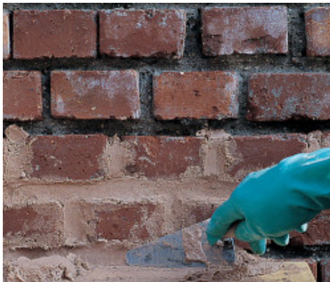
Pointing a brick work using Mape-Antique CC
