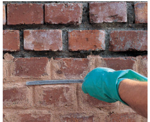
Finishing the joints pointed with Mape-Antique CC
