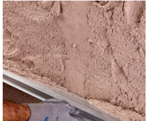
Flattening the surface of Mape-Antique CC with a straight edge
