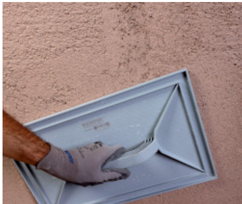
Levelling the surface of Mape-Antique CC
