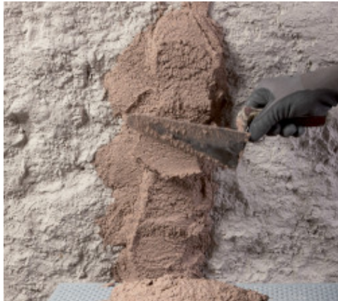
Preparation of levelling strips
