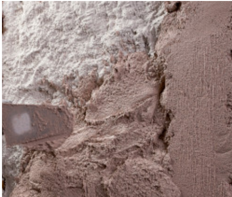
Application of Mape-Antique CC over Mape-Antique Rinzafo
