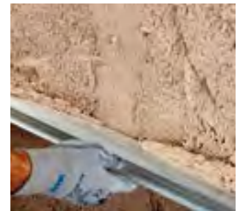
Compacting the dehumidifying render with a straightedge
