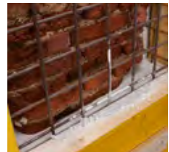
An area of the masonry mortar after pouring
