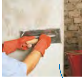
Spreading a transpirant, smooth texture skim coat
