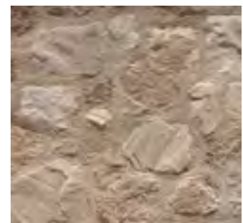
Reconstruction of a stone facing wall
