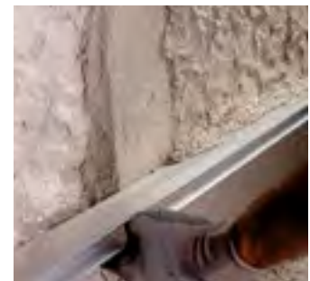
Compacting the dehumidifying render with a straightedge
