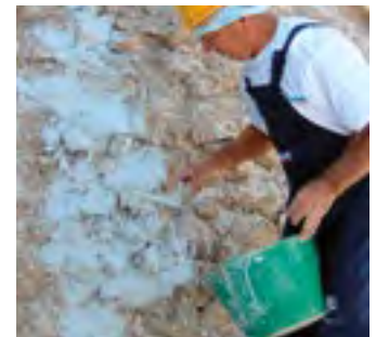
Application of a scratch-coat layer by trowel
