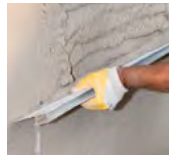
Compacting the transpirant render with a straightedge
