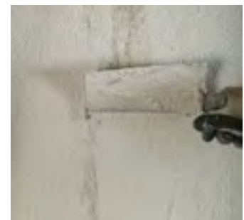
Application of dehumidifying render
