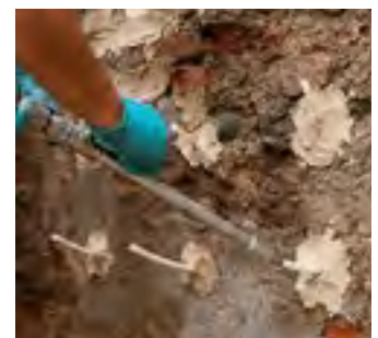
Injecting Mape-Antique I-15
