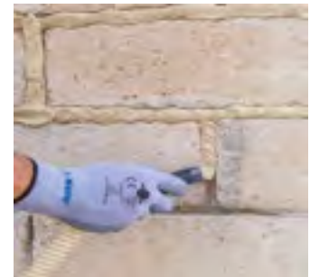
Building stone masonry
