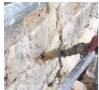
Consolidation of “rubble masonry” stone masonry
