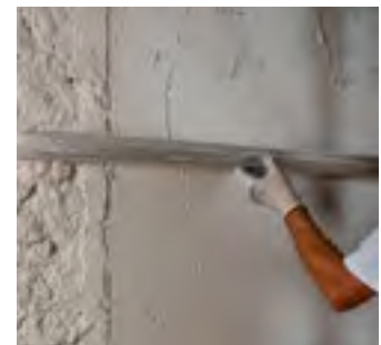
Compacting the dehumidifying render with a straightedge
