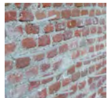
Consolidation of a brick parapet wall
