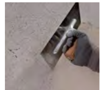
Application of coarse texture skimming mortar
