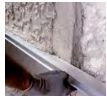
Compacting the dehumidifying render with a straightedge
