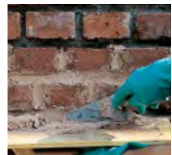
Pointing between brickwork
