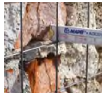
Checking the gap between the mesh and substrate
