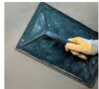
Levelling off the transpirant render
