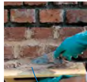
Pointing between brickwork
