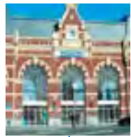
Cambrai Railway Station - France
