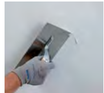
Application of the second layer of ultra-smooth texture skimming mortar
