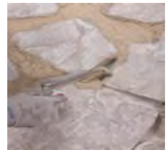
Pointing “exposed” masonry
