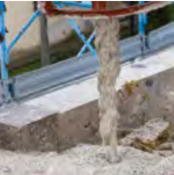
Casting mortar into formwork
