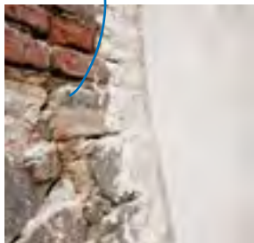
Dehumidifying render mixed on site
