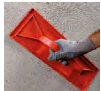
Levelling off the dehumidifying render
