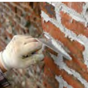
Pointing between brickwork
