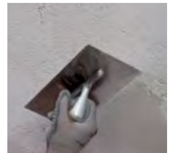
Application of fine texture skimming mortar
