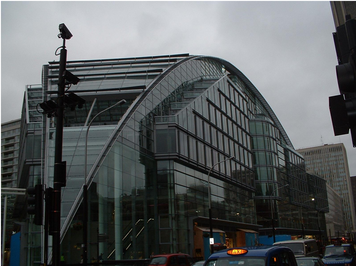
Above: A front view of cardinal Place near Victoria Station in London
