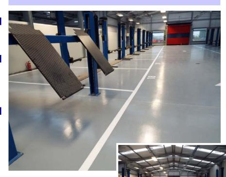
was selected as a high quality, damp tolerant resin, with a wide application spectrum and VOC free properties. ADD 250 Polymer Beads were then added to provide an anti-slip, textured finish to give a surface that remained easy to clean.
