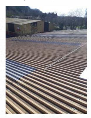
Tape Application - Where Required Apply Noxyde Tape centrally over the joint detail, pressing firmly into the profile of the panel avoiding stretching, tenting or creation of any air pockets. Ensure that the Noxyde Tape is well adhered to both surfaces.
