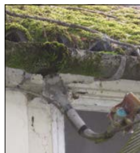
Moss and lichen growth on AC roofing and gutters
