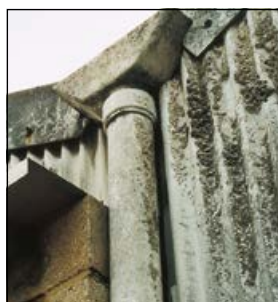
Moss and lichen growth on AC roofing and gutters
