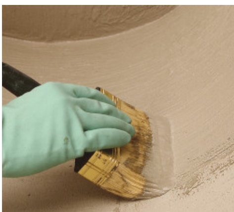
Waterproofing of details by brush
