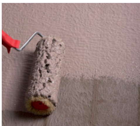
Waterproofing of details by roller
