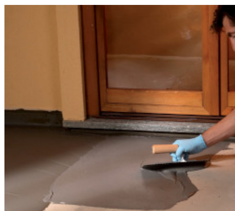
Waterproofing of terraces by trowel
