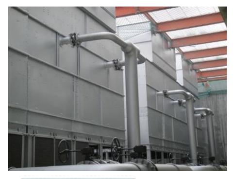
System:Sandblasting SA 2.5 on old hot-dipZINGA1 x 60 μm DFTALU ZM1 x 50 μm DFT
