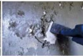
Stripping off coating
