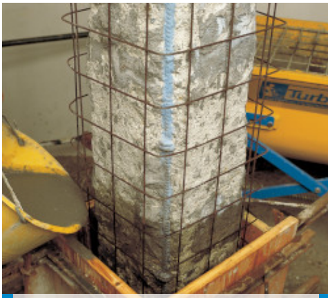
Pouring into a formwork
