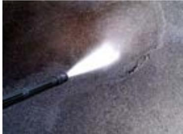
**Clean the surface thoroughly using a jet wash**
