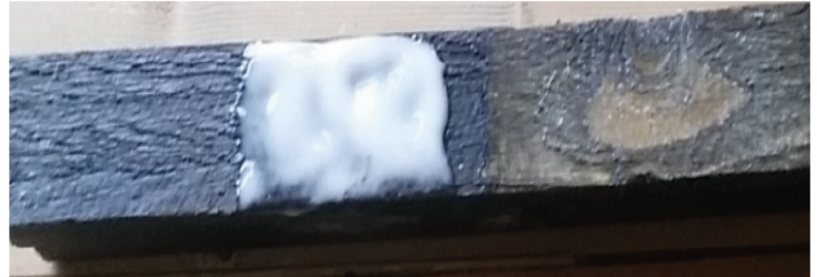
Painted wood surface • Paint Stripper applied • Wiped off and paint removed
