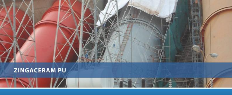
A very hard-wearing and UV-resistant acrylatepolyurethane topcoat that has been pigmented with ceramic particles to prevent erosion of the surface from wind-blown sand and dust particles.
