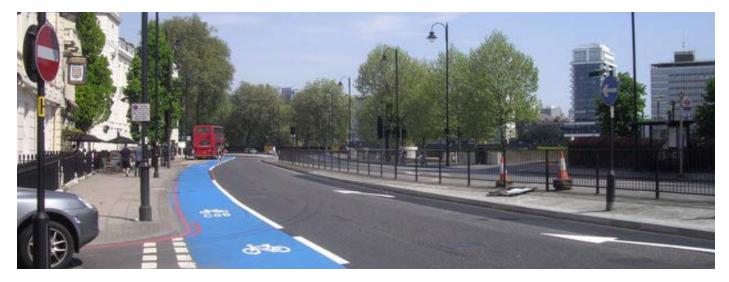
A recent project completed using preformed thermoplastic markings was Cycle Superhighway CS5 running from London Vauxhall to Victoria.
