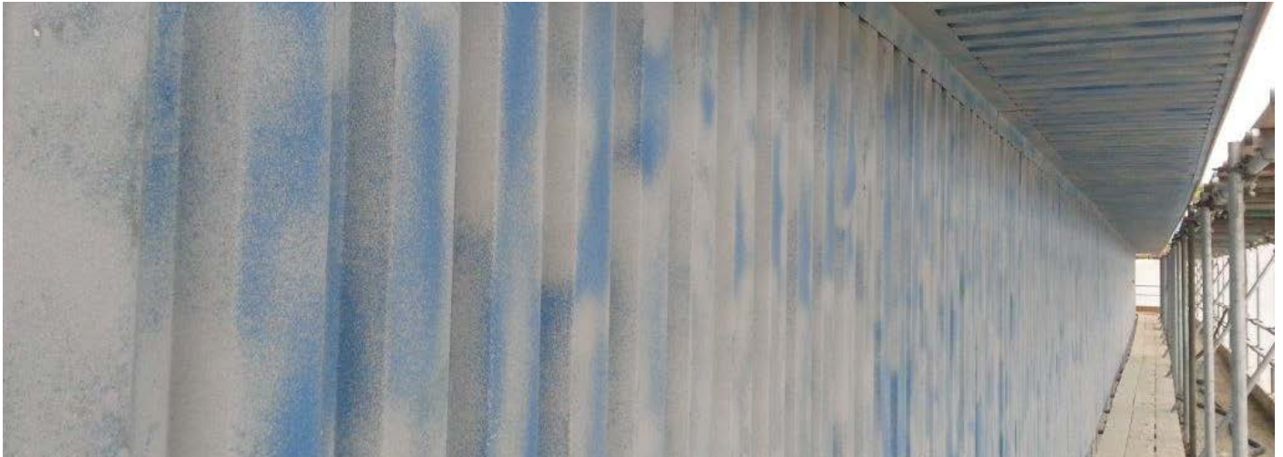
After Sweep Blasting
