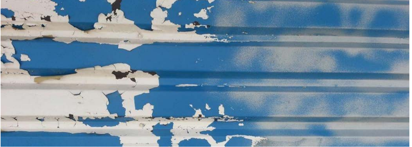
Before Sweep Blasting
