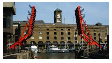
Promain offered 2 systems the first being to sand blast the steelwork apply a coat of PPG Amerlock 2, a two pack moisture tolerant epoxy followed by a coat of Sigmadur 550, a high gloss chemical and UV resistant polyurethane topcoat.
