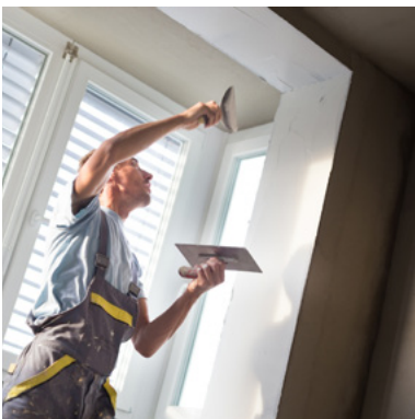
Protection during plastering
